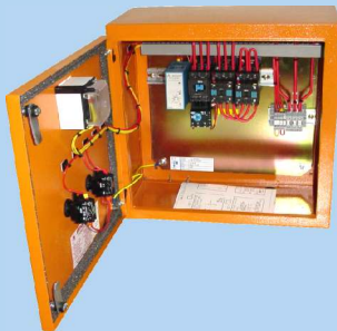
ENCLOSED STAR DELTA STARTER
